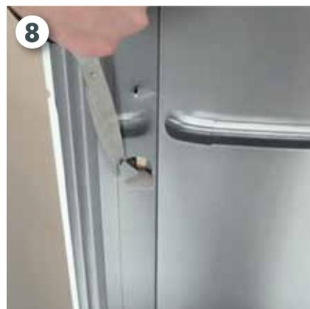
Mark the position of the door handle and cut an aperture for it
